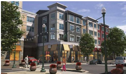
Figure 25 Mixed Use Housing Examples – Rhode Island Avenue Development and Kirkland Juanita Village
