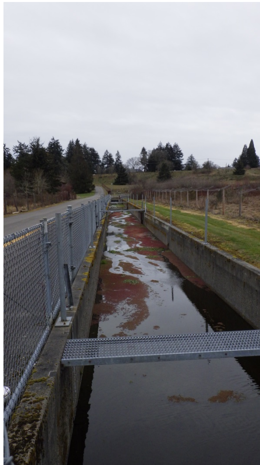
Spring-fed creek in concrete channel, Lakewood hatchery grounds (27 Feb. 2019)
