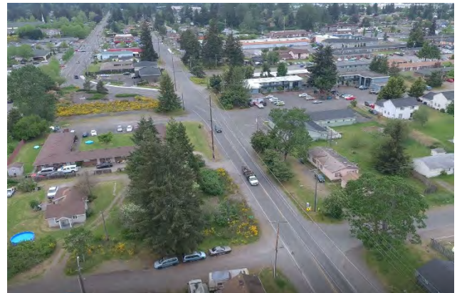
111 th and 112 th Street Corridors
